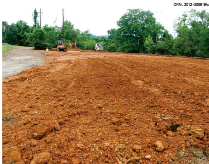
Fig. 3.25. Placement of clay layer over exposed coal ash.
