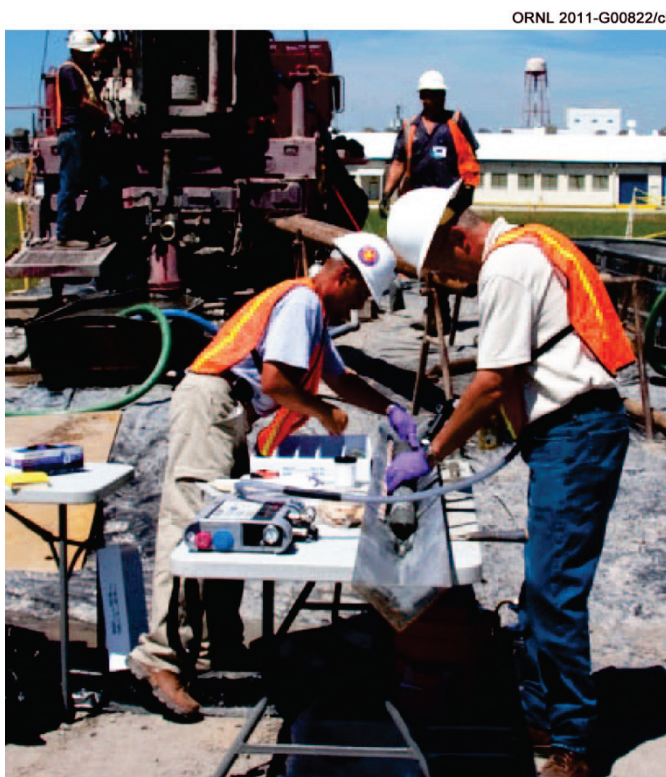
Fig. 3.71. Drilling exploratory boreholes near the K-1401 area.
