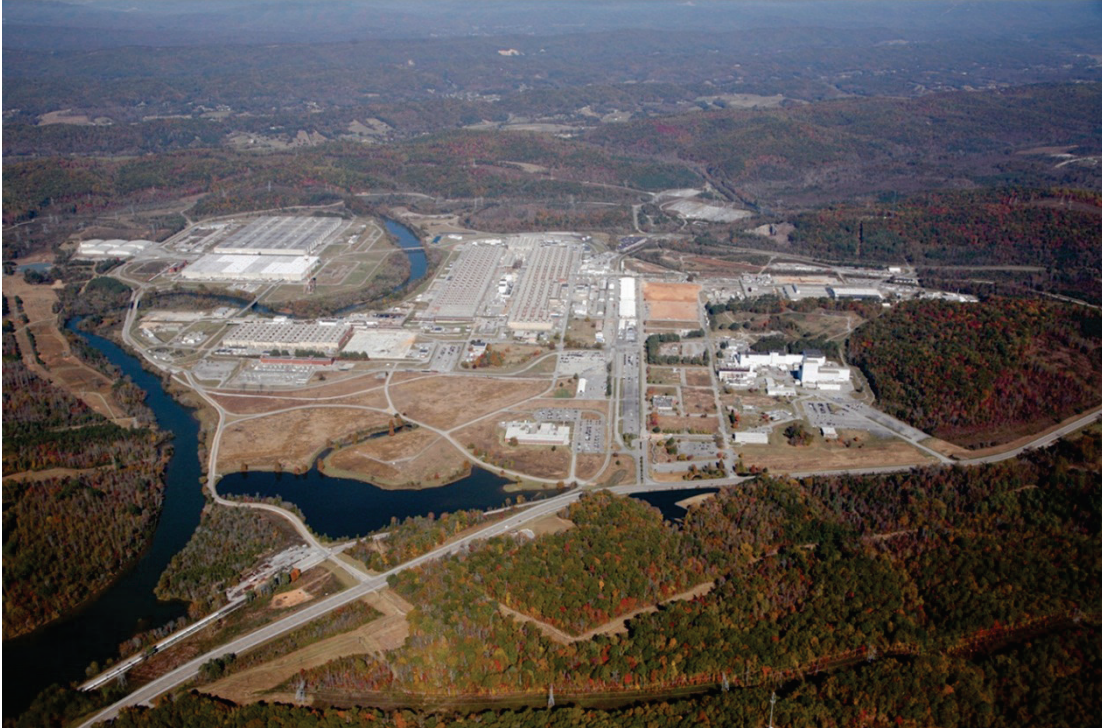
Fig. 3.1. East Tennessee Technology Park.
