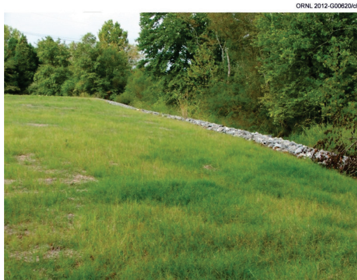
Fig. 3.26. Ash pile area after remedial actions were completed.
