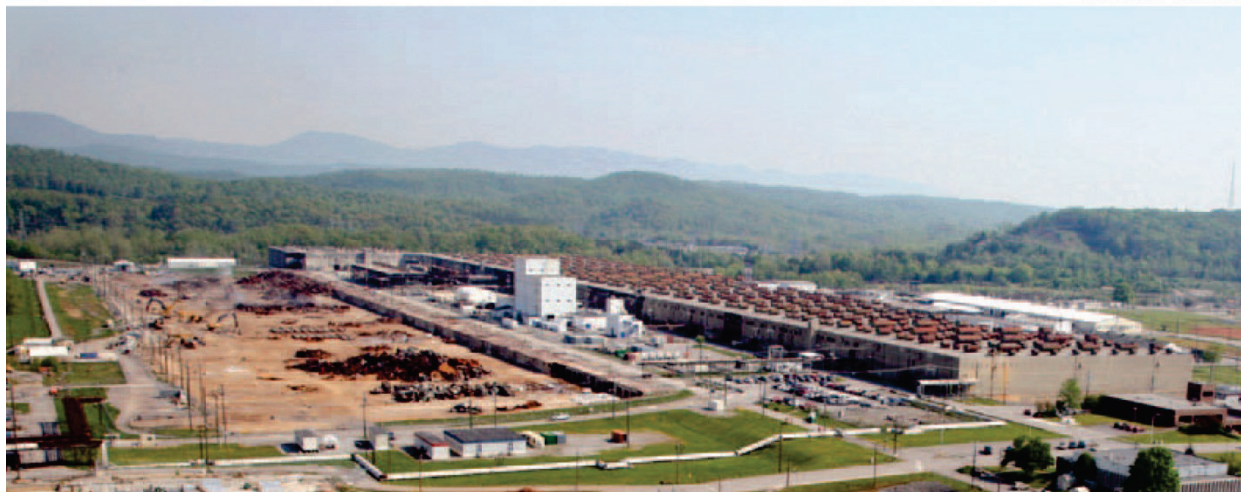
Fig. 3.70. The K-25 Building after demolition of the west wing.
