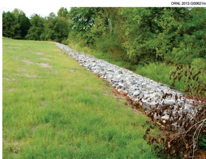
Fig. 3.27. Completed placement of rip-rap along bank of ash sluice channel.
