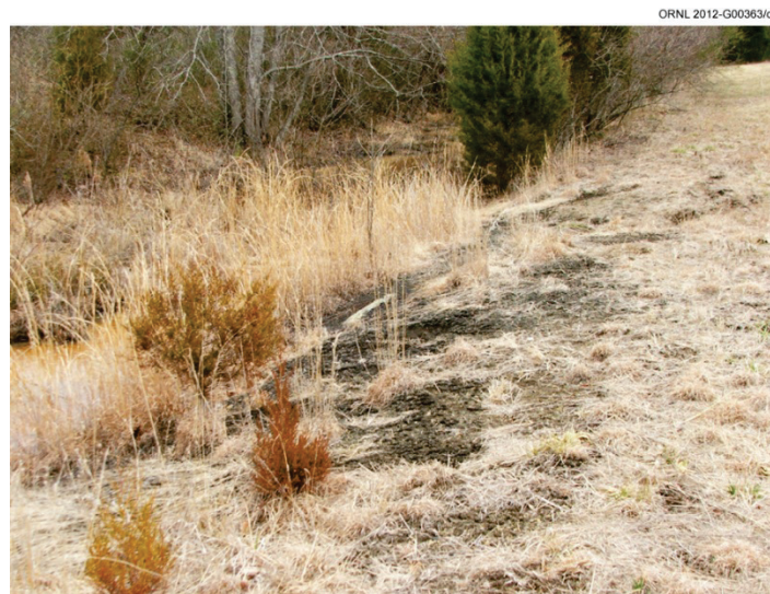
Fig. 3.22. Exposed ash near ash sluice channel.
