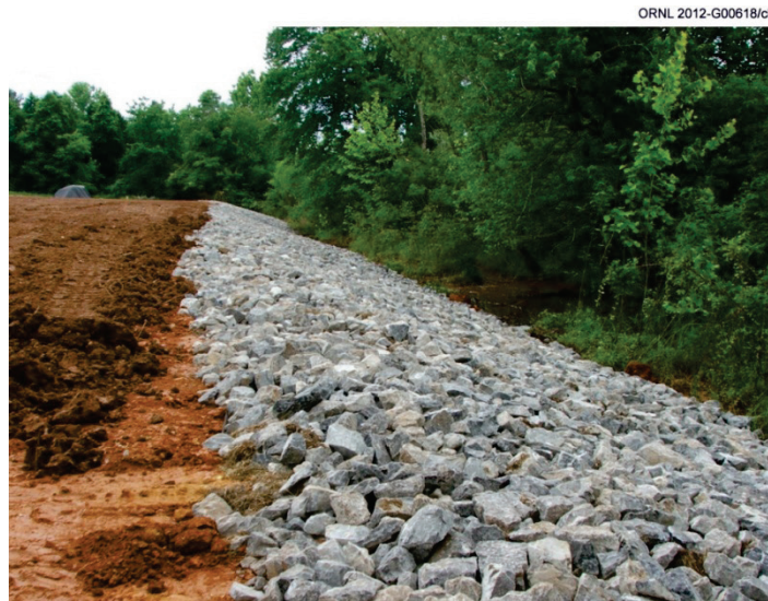
Fig. 3.24. Initial installation of rip-rap along bank of ash sluice channel.
