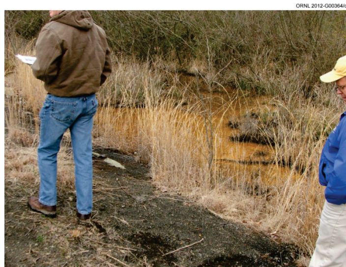
Fig. 3.23. Another area near ash sluice channel where ash had not been properly covered with soil.
